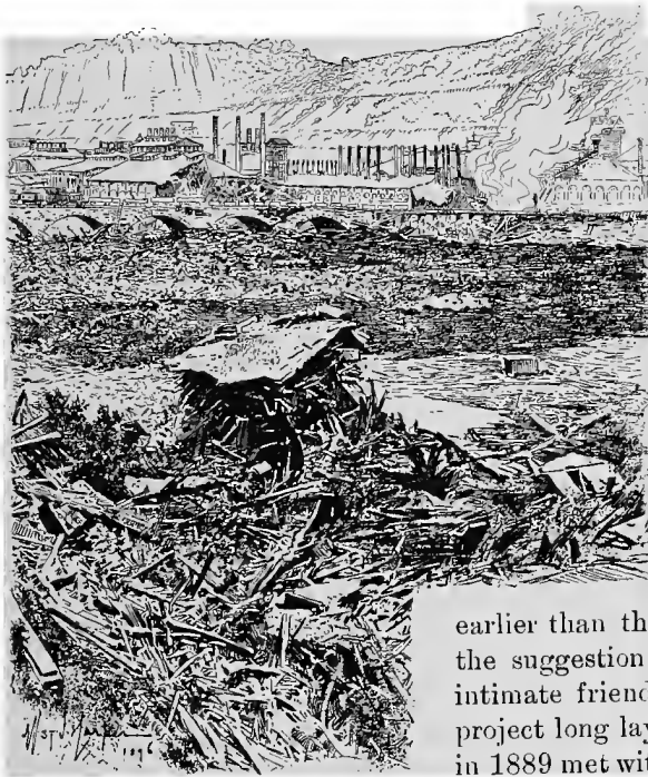
The Great Drift and the P. R. R. Bridge after the Flood.
